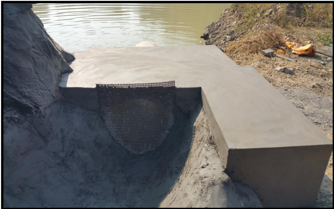
Slit trap to prevent quarry wastes entering in to the main stream
