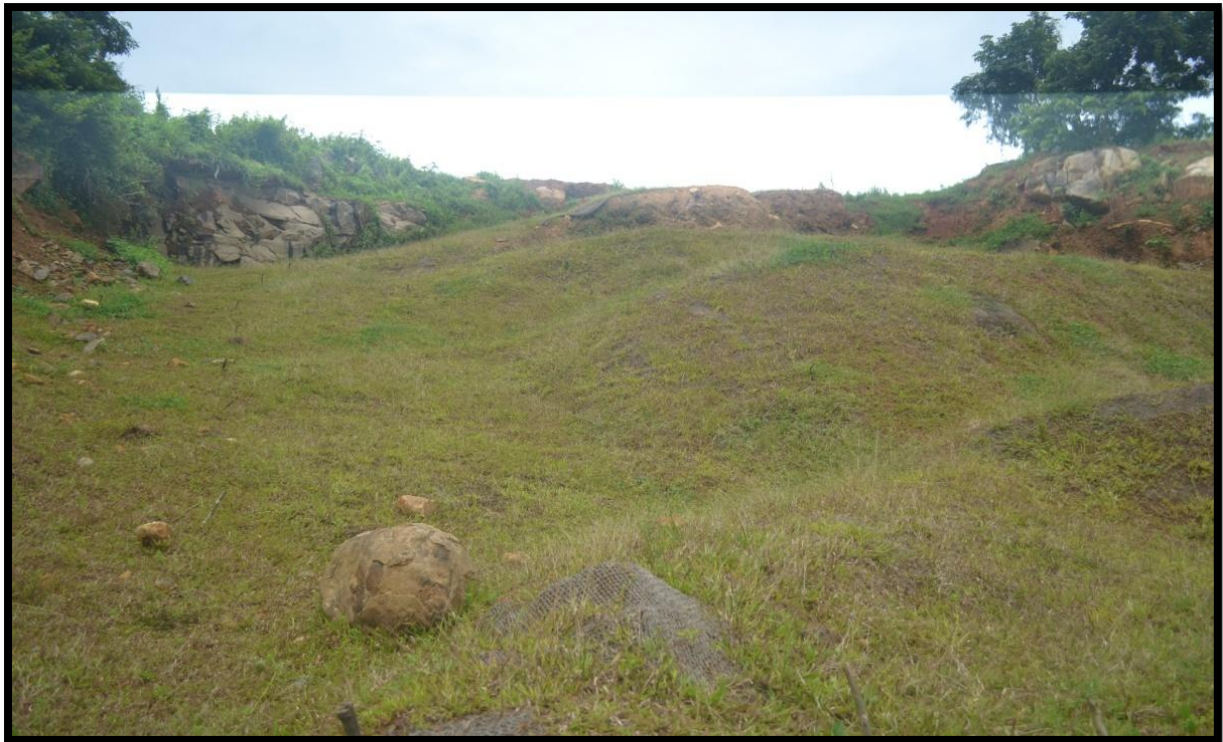
Benches made by over burden and covered by coir mat
