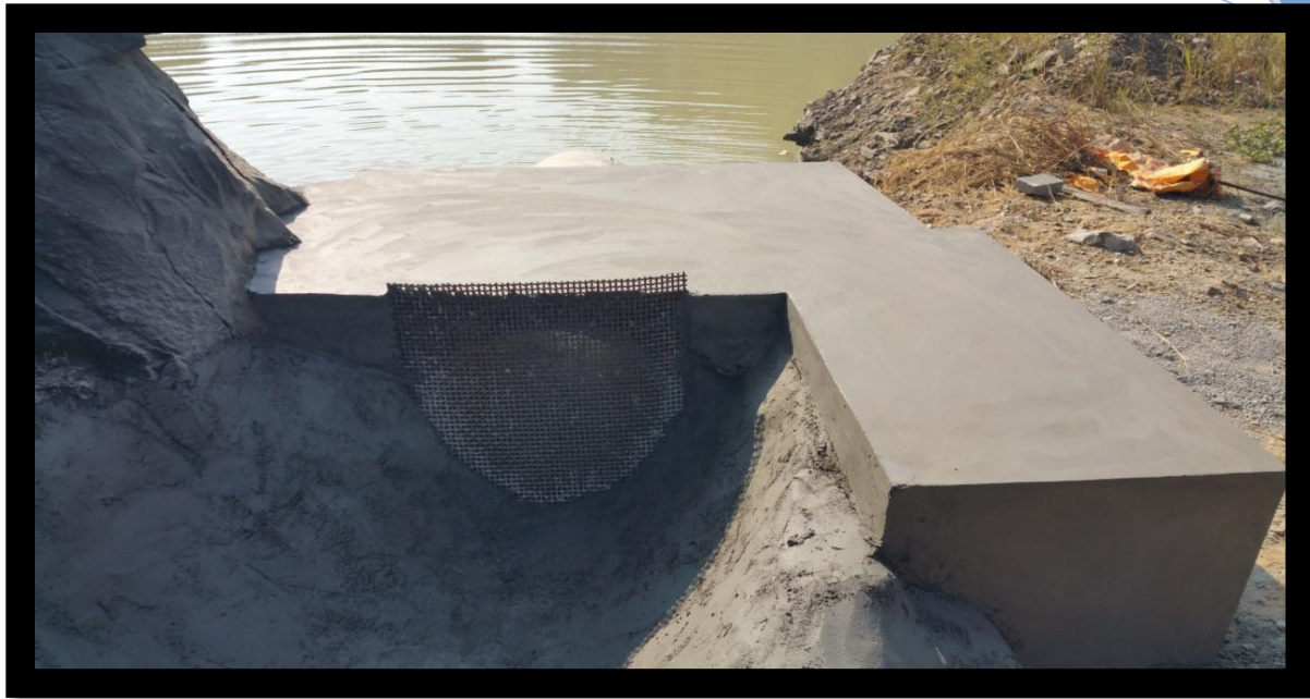
Slit trap to prevent quarry wastes entering in to the main stream
