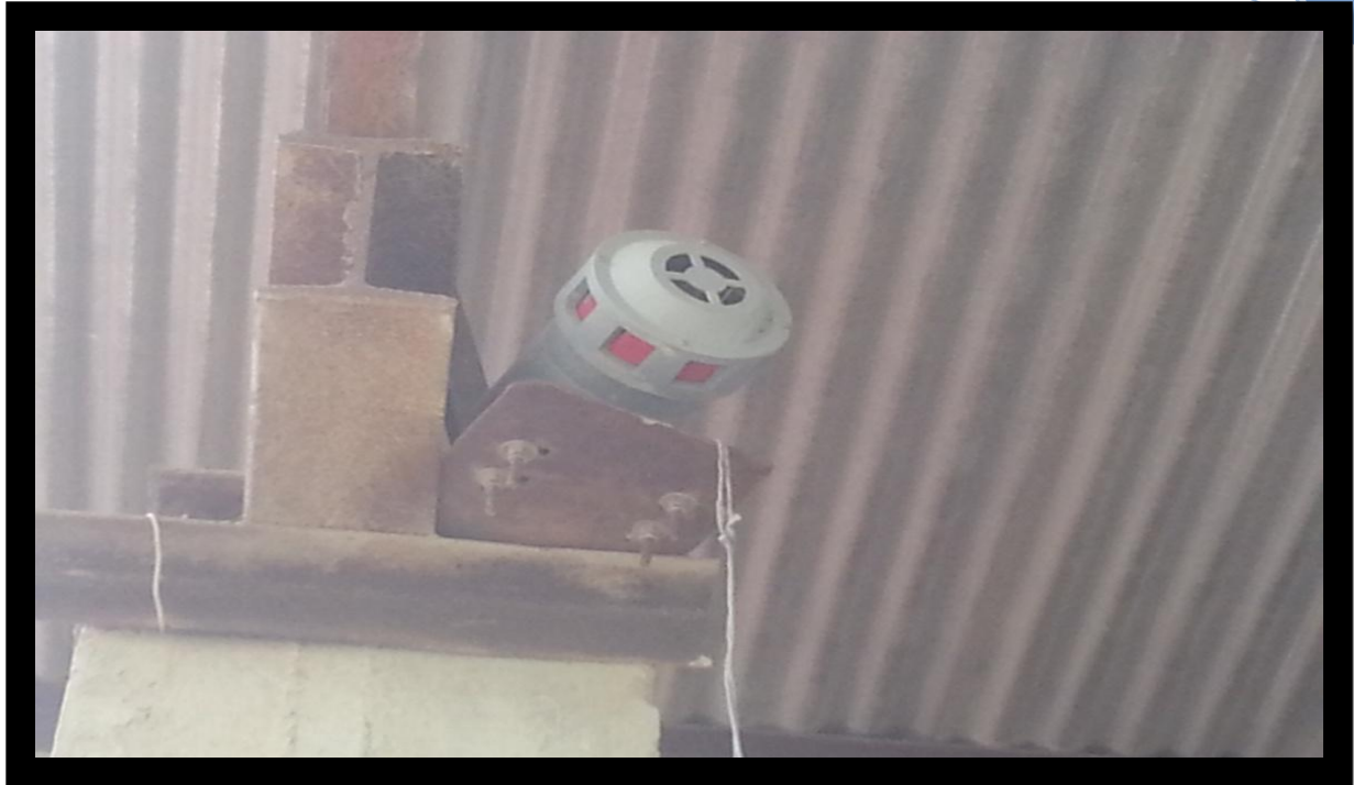
Device for alarm prior to the blasting
