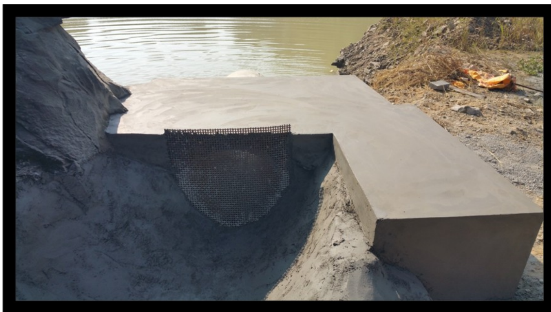
Slit trap to prevent quarry wastes entering in to the main stream
