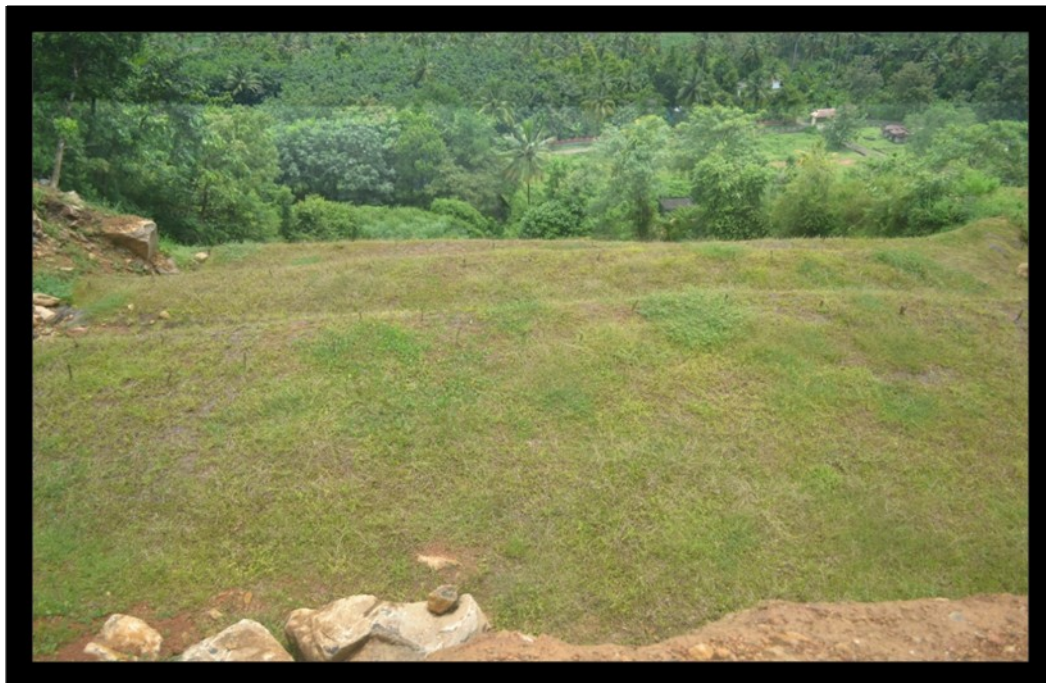
Benches made by over burden and covered by coir mat
