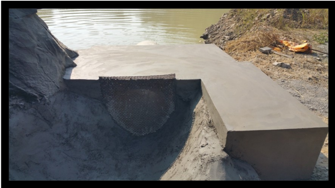
Slit trap to prevent quarry wastes entering in to the main stream
